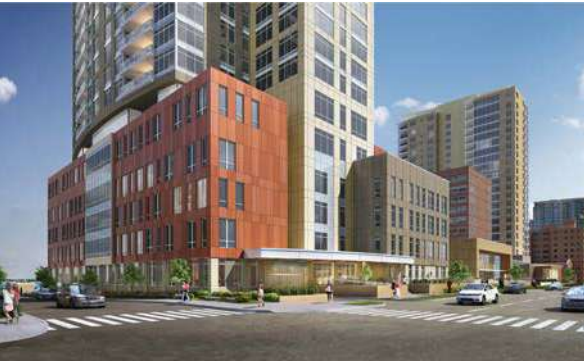
Saint John's On The Lake Newest tower addition to open in 2020
